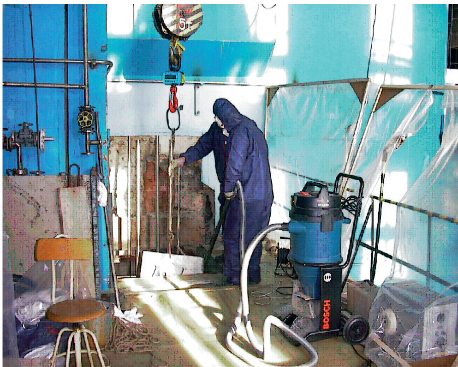
FIG. 5. Decontamination activities during refurbishment of the SRR's spent fuel pool.
